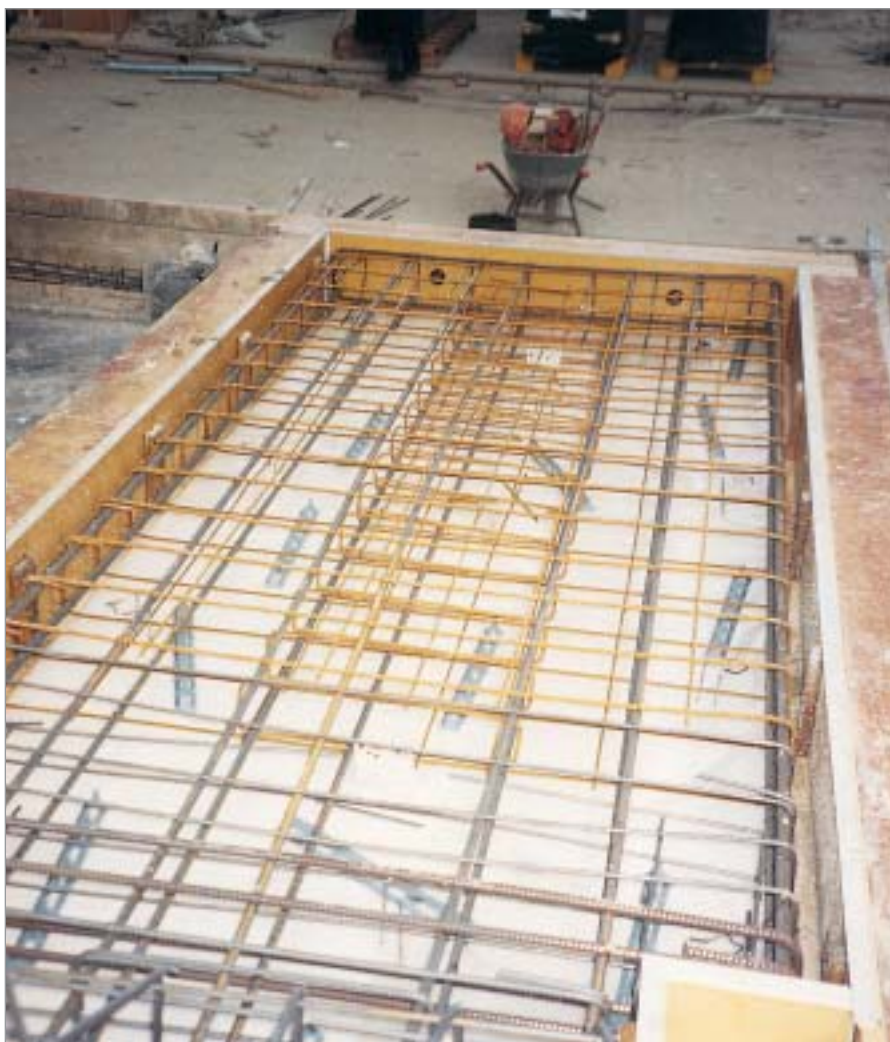
Formwork with coated glass panel and reinforcement in place
