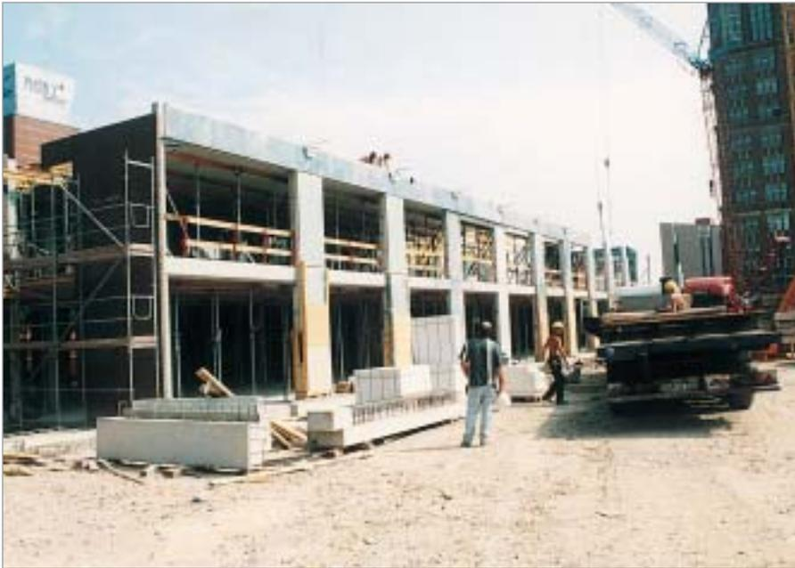
**Installation of a monolithic element – façade and load-bearing structure as a single unit**
